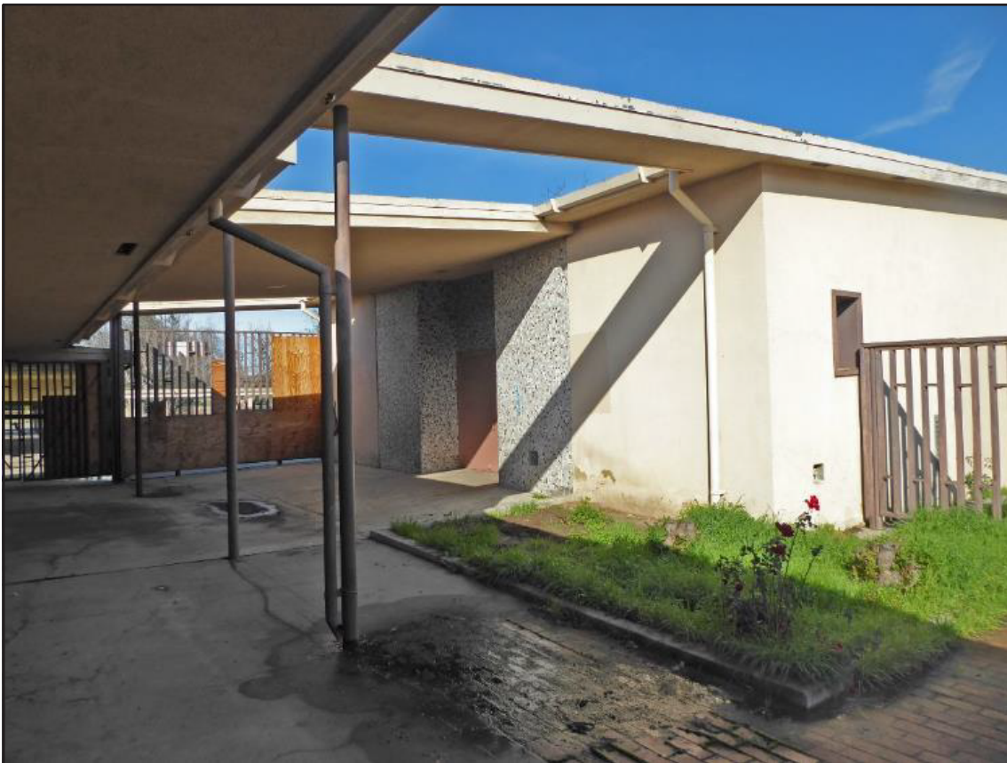
View looking northwest at the main entrance to the school, with the Main Building on the left and the Multi-Purpose Building on the right.
