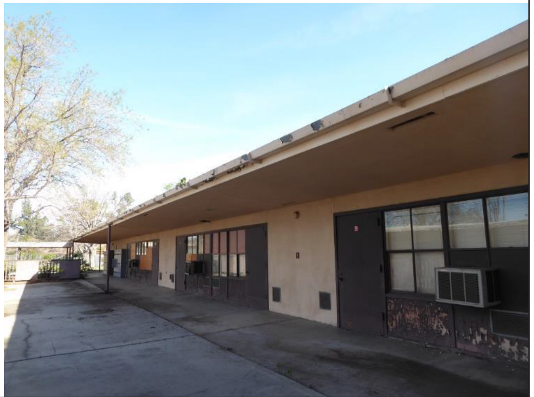
View looking northeast at the west façade of Classroom Building A.
