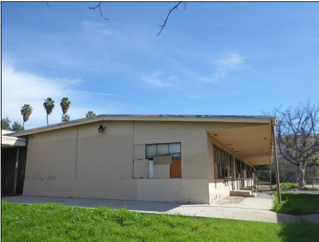
View looking northeast at the west and south façades of the Main Building.
