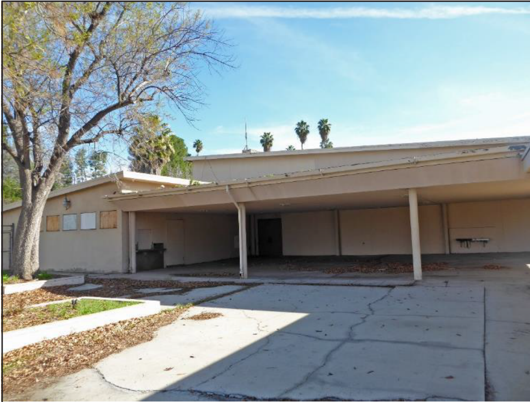
View looking northeast at the lunch pavilion, with the two wings of the Multi-Purpose Building to the rear.
