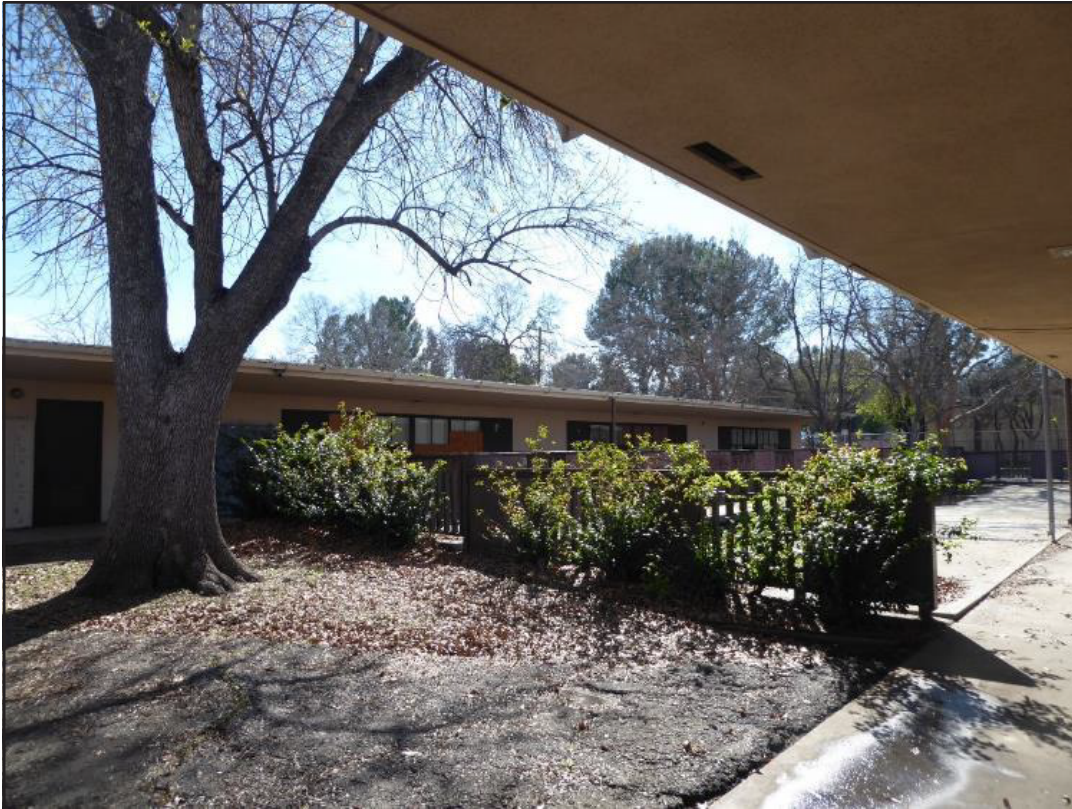
View looking southeast at the west façade of Classroom Building A.
