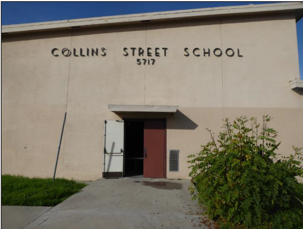
Detail view of the entrance on the east façade of the Multi-Purpose Building.
